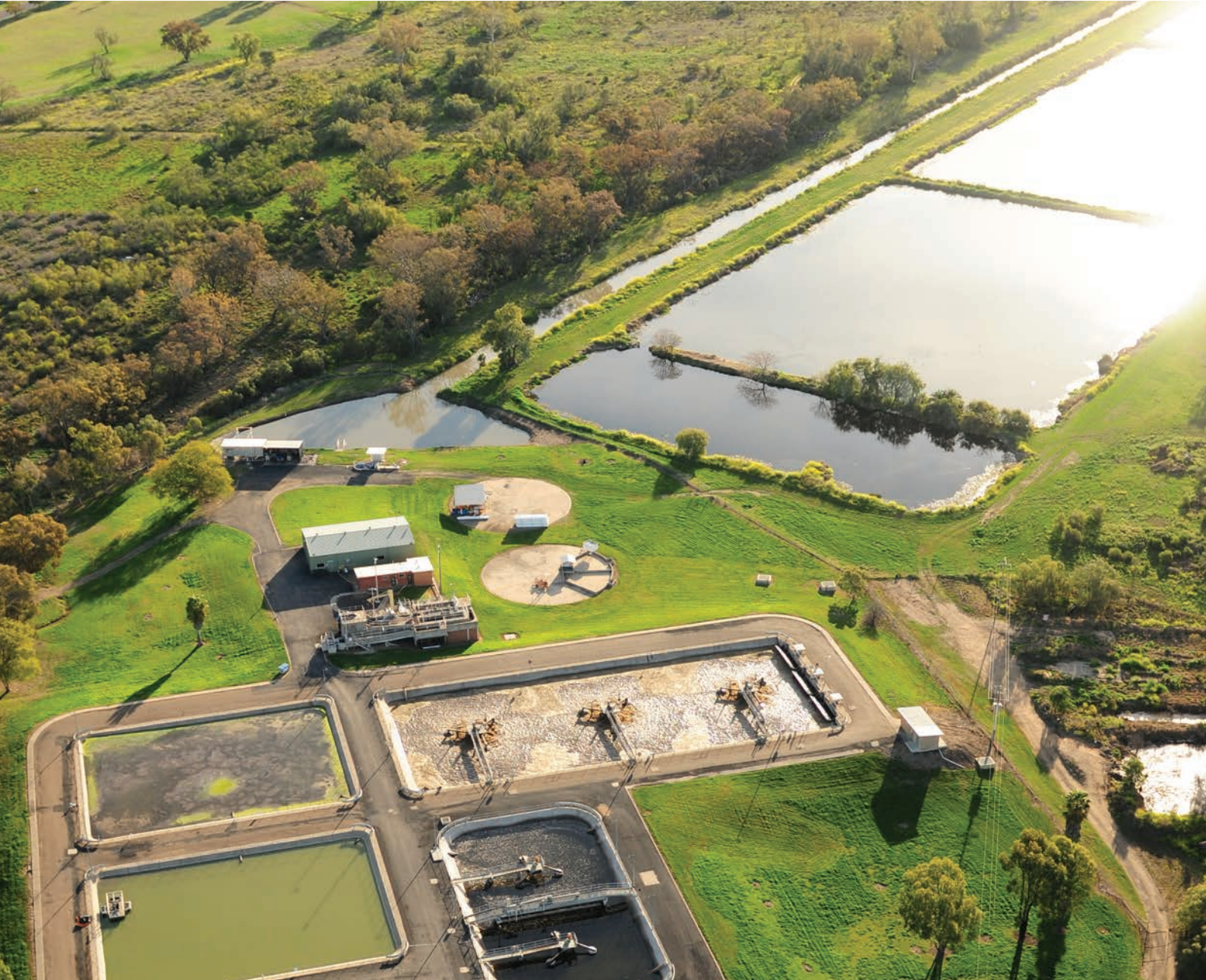
Moree Sewerage Treatment Plant
