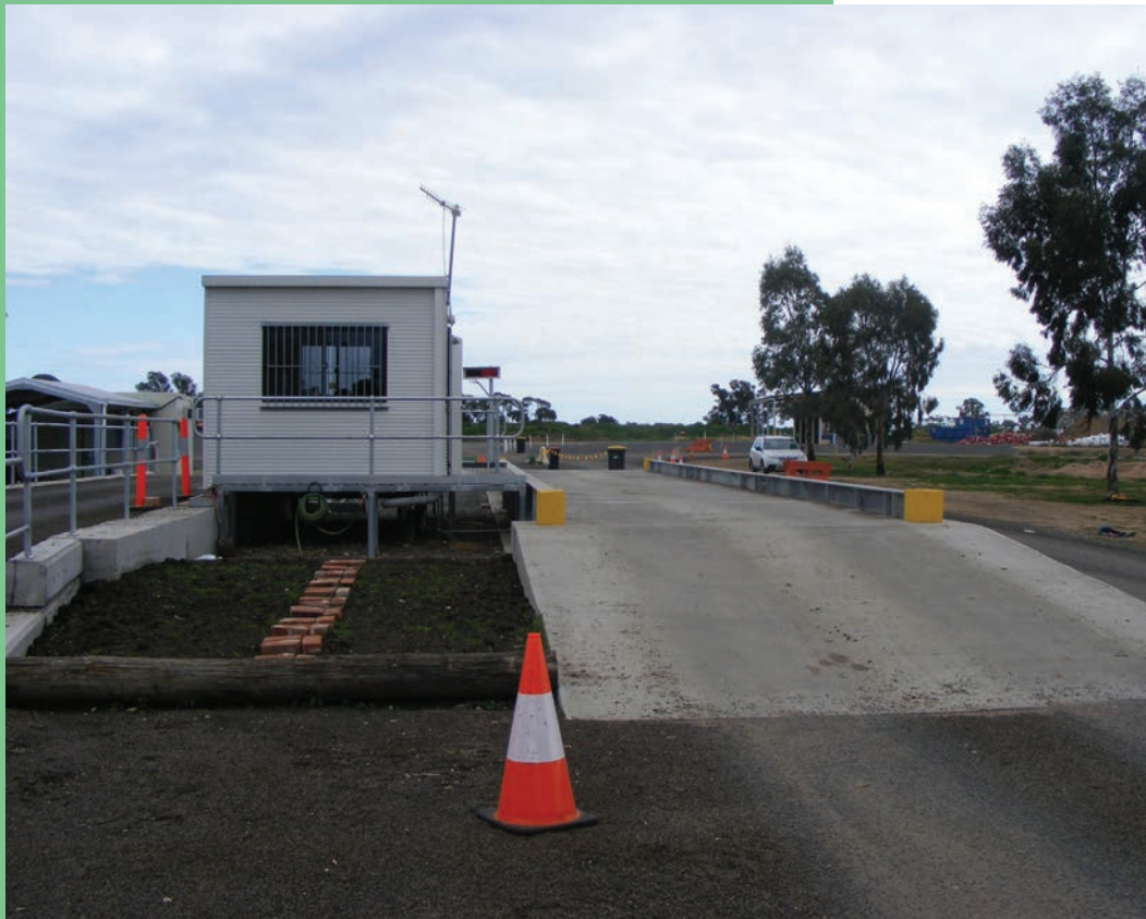
Narrabri landfill facility today (Peter Cotterill)
