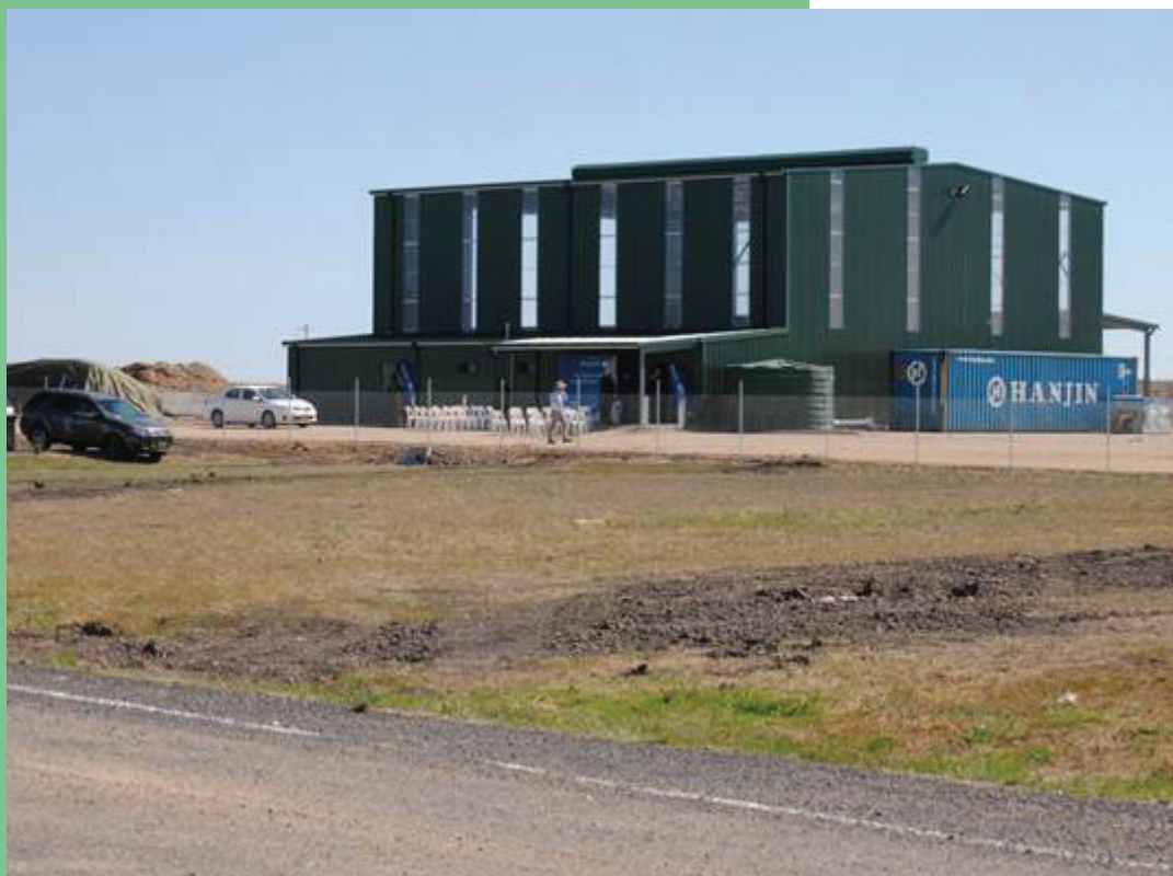
Cleanaway Recycling Shed and the Organics Waste Depot
